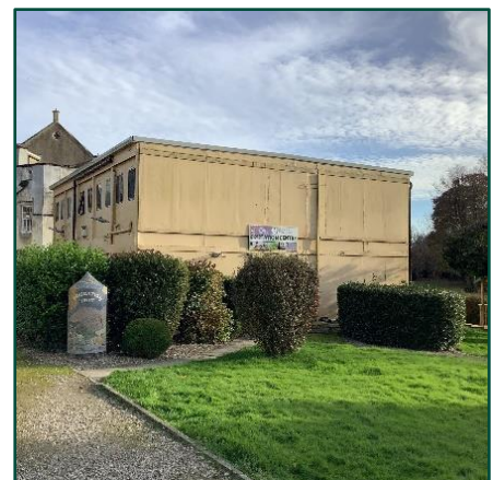
Figure 11: Education Centre Building, Shelton Abbey
